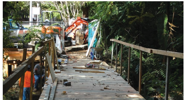
Photos from top, right: Fern Dell completed pedestrian bridge. Note how the arch is repeated on both bridges. Middle: Recently installed black fencing and signage. Bottom: Bridge during construction phase. Left side: Postcard showing 1930s-era bridge.
