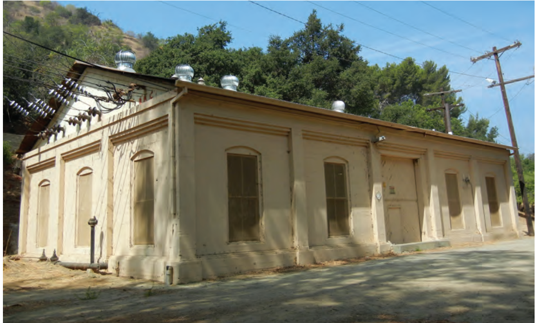
LADWP power house located near the Crystal Springs Picnic Area.
