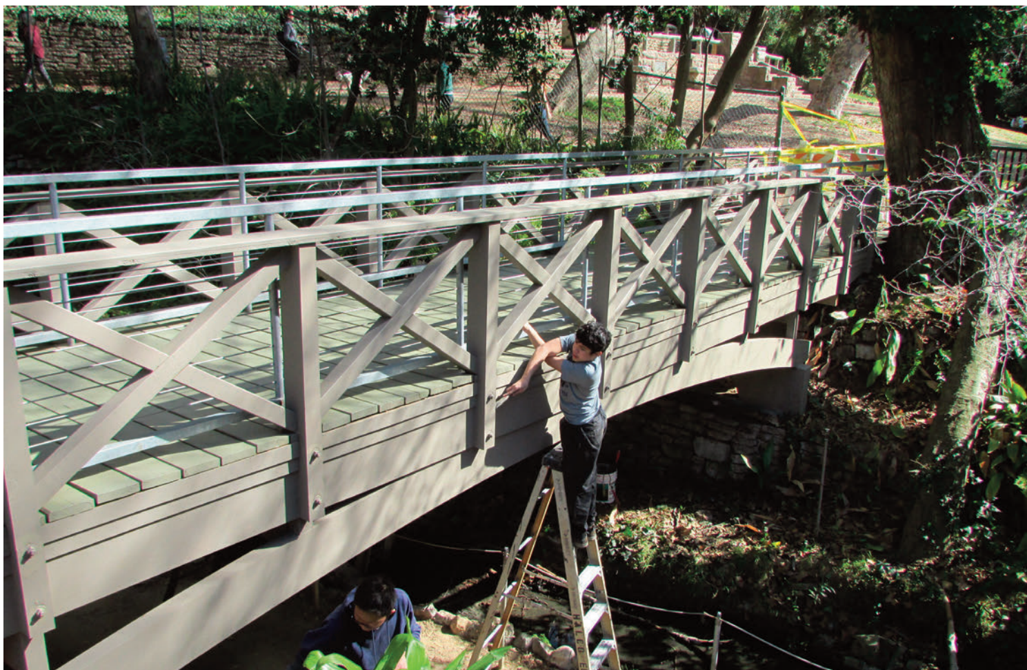
Applying finishing touches to bridge hardware.
