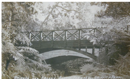
A bucolic view of the pedestrian bridge surrounded by ferns from the 1930s.
